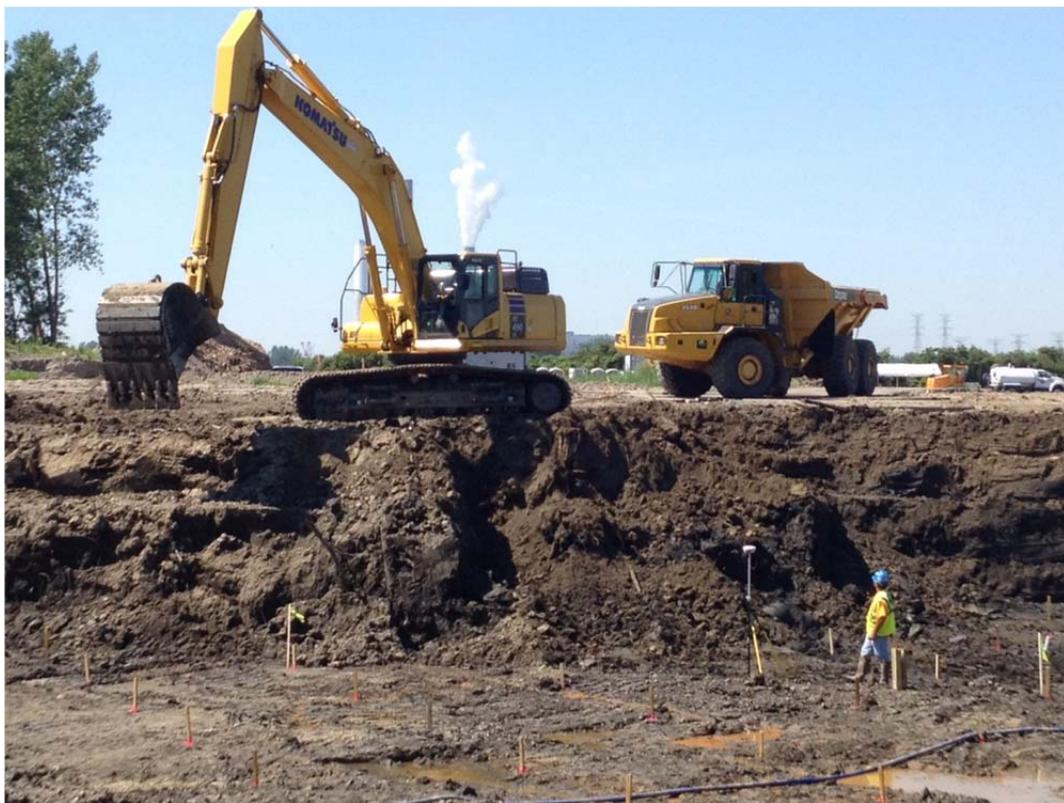
**Photo 1. Excavation of existing materials from confined disposal facility.**
