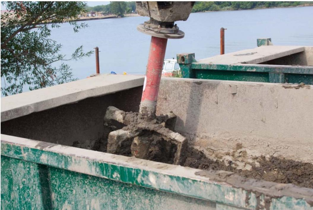
**Photo 3: Backhoe-mounted custom paddle to blend Portland cement with sediment.**
